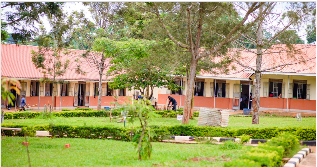
Some of the Classroom blocks
